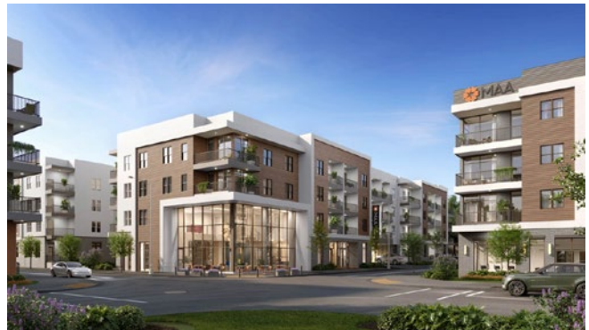
RTP’s first apartments, MAA Nixie, opened at Hub RTP in October 2024.
