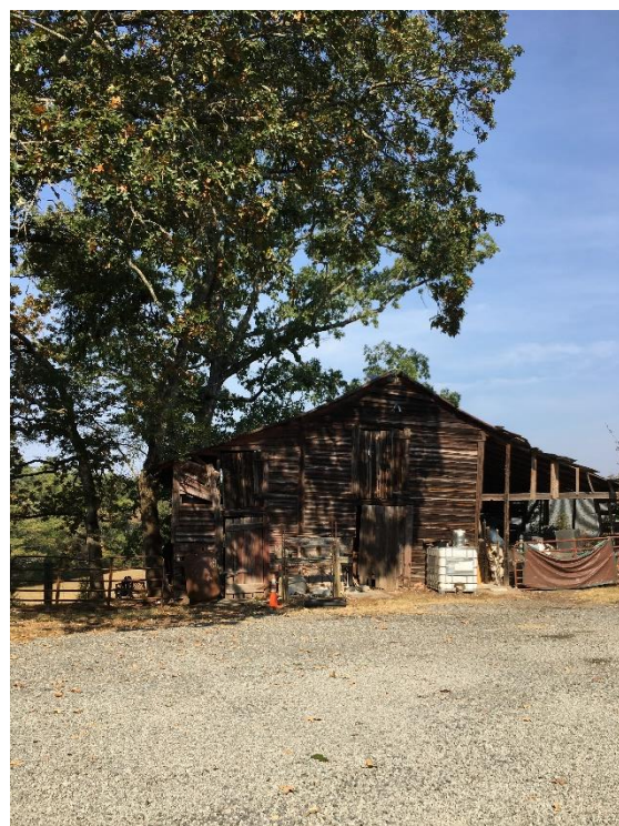
One barn located on farm along Herndon Rd
