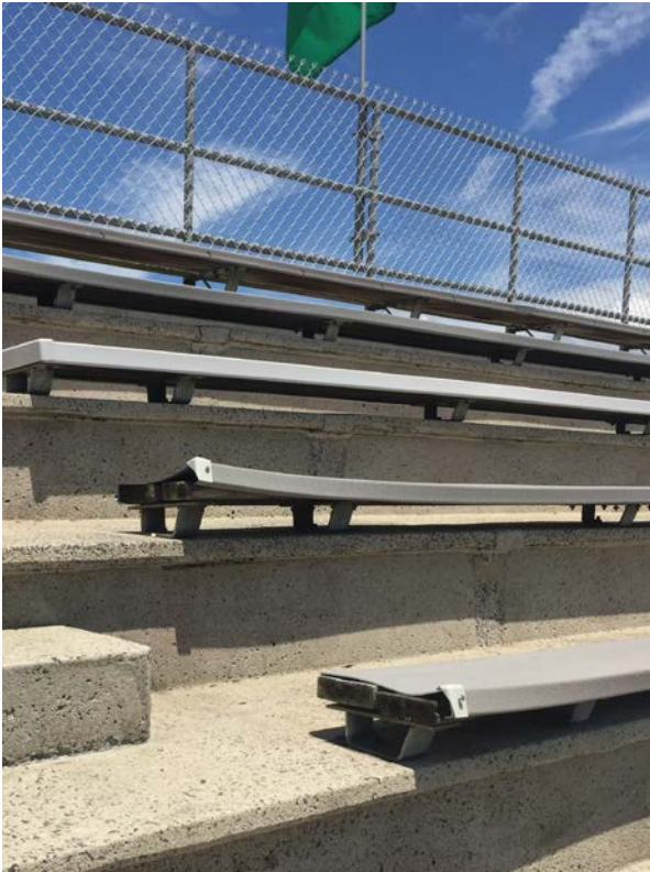
Current Stadium Seating
