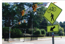
User-activated stop light (Pedestrian Hybrid Beacon)
