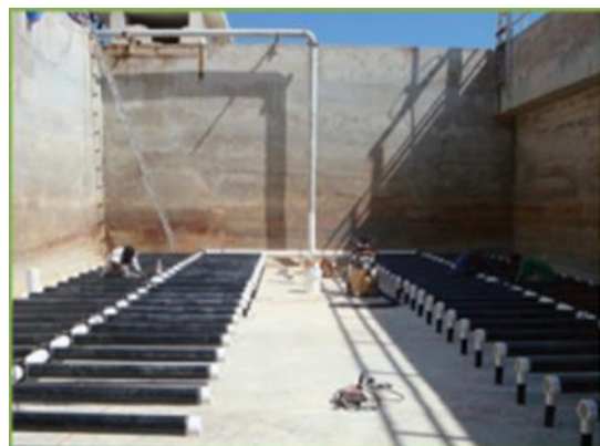
Figure 3-3: Tube Diffusers
