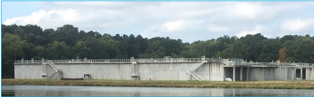
Figure 1-1: TWWTP BNR Treatment Trains
