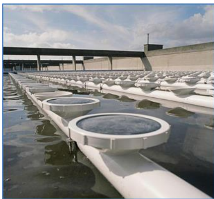
Figure 3-2: Membrane Disc Diffusers
