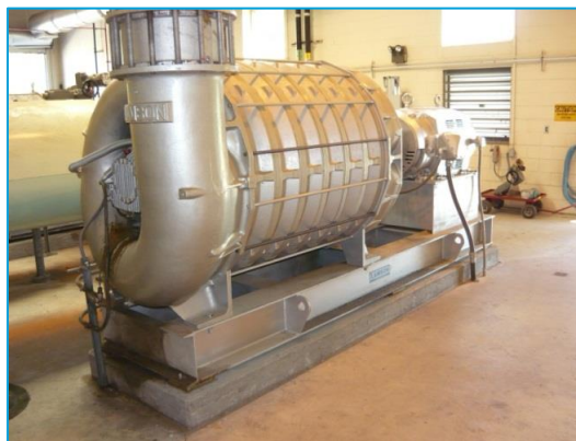
Figure 3-8: Typical Multi-stage Centrifugal Blower
